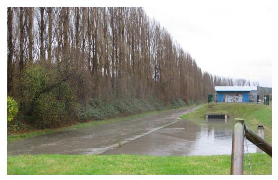
Figure 18 Overflow event at CSO facility Wörthstraße discharging into the upper Emscher (photo: Jörg Rothholz)
